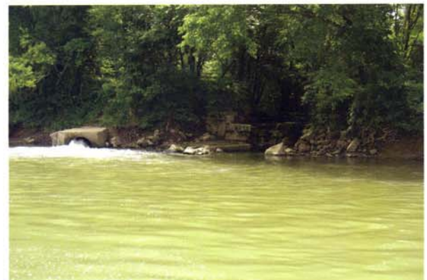
BGMU outfall on Barren River
